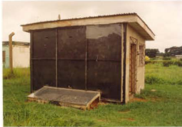
Fig. 1: Trombe wall poultry chick brooding house
